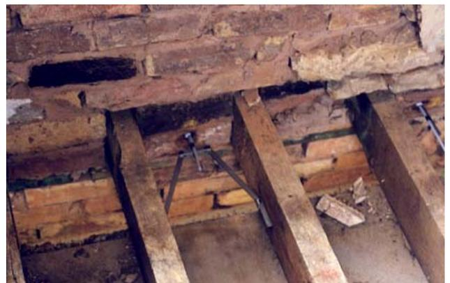
Can be used as a “through building tie” by placing at each end of joists with “double Armlock” connection if joists are lapped.
