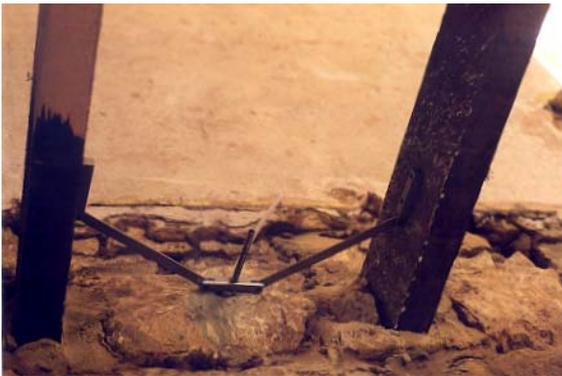
The “Armlock” is connected to the wall by an embedded stud fixing (Not included) and easily adjusts to the joist spacing.
